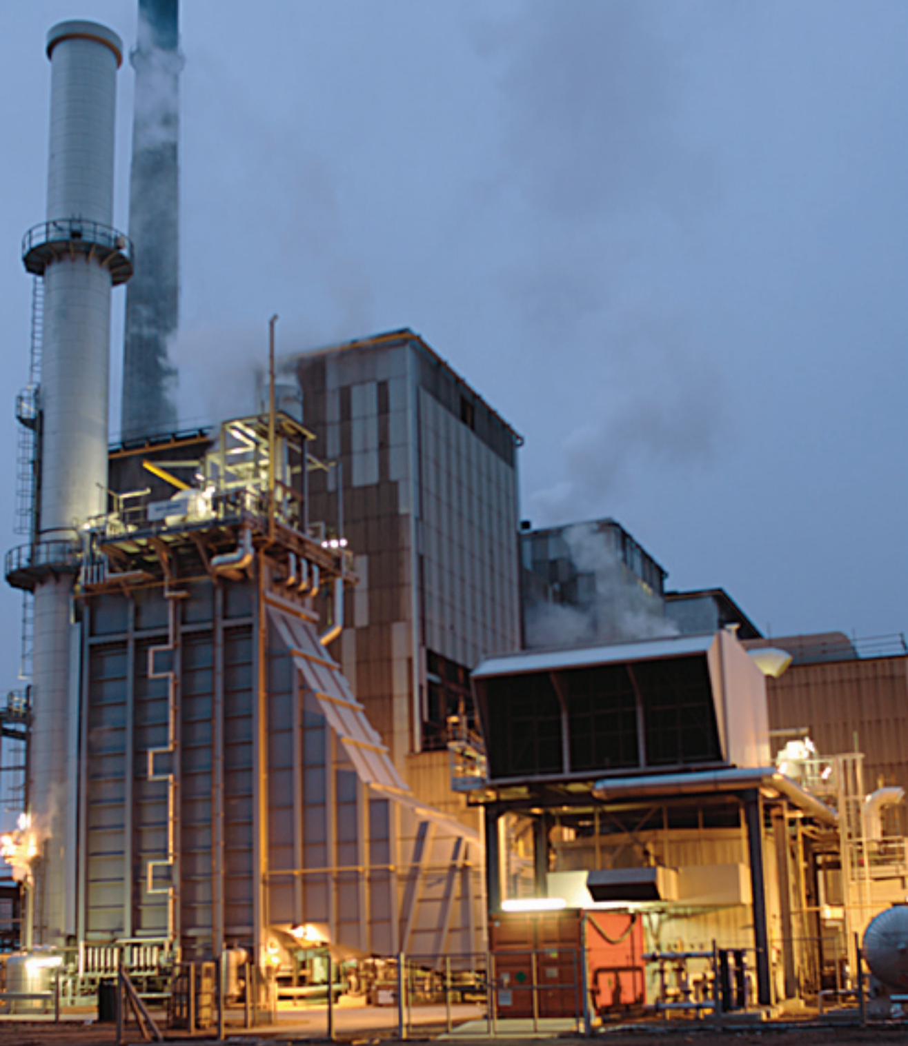
SembCorp Utilities UK's new gas turbine (pictured) has increased electricity output at the Wilton Power Station and at the same time added to the fuel flexibility and environmental efficiency of our operations.
