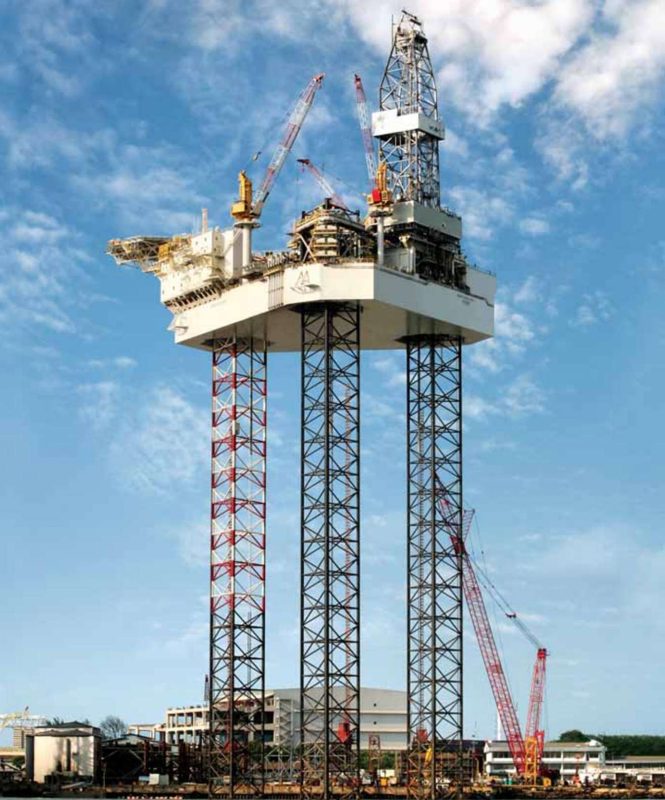
Jack-up rig built by SembCorp Marine's shipyard in Singapore
