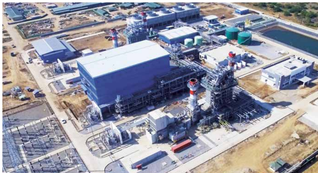
When fully operational, the 225-megawatt gas-fired Sembcorp Myingyan Power Plant will help to ease Myanmar's power deficit
