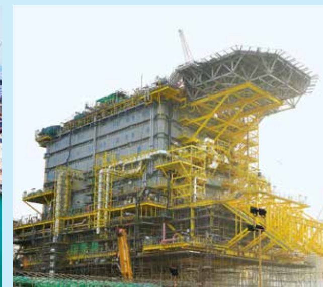
One of three topsides under construction for Maersk Oil. On completion, the topsides, comprising a central processing facility plus two connecting bridges, a wellhead platform and utilities and living quarters platform, will be installed in the Culzean field in the UK North Sea
