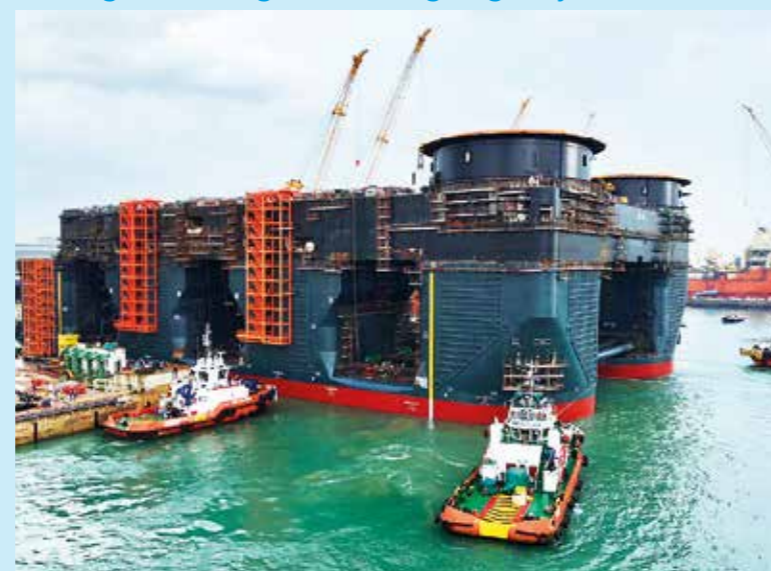
Measuring 220 metres by 102 metres, the 273,700-metric tonne semi-submersible crane vessel Sleipnir , currently under construction at our yard for Heerema Offshore Services, is the largest in the world
