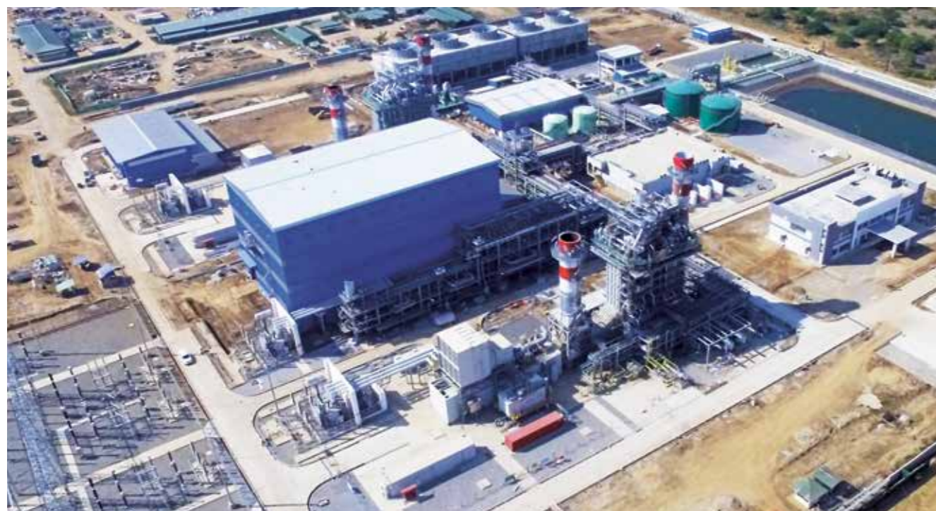
When fully operational, the 225-megawatt gas-fired Sembcorp Myingyan Power Plant will help to ease Myanmar's power deficit
