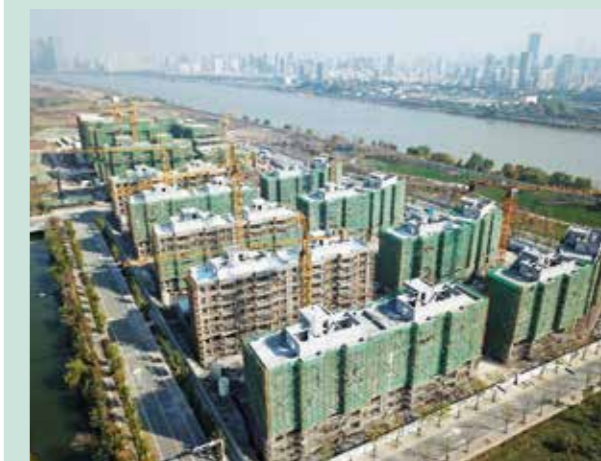
International Water Hub in China, a technology and business centre, as well as Riverside Grandeur, a residential development next door, celebrated their topping out in 2017. Both projects are on track to be completed in 2018
