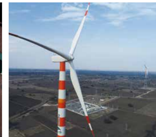
Commenced commercial operations of the 250-megawatt SECI 1 wind power project, the first to be delivered under India's nationwide wind power tenders
