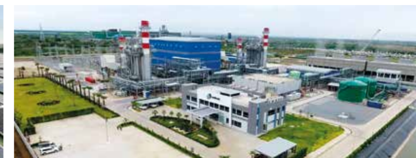
Commenced full commercial operations of Sembcorp Myingyan Independent Power Plant, a 230-megawatt combined cycle gas-fired power plant in Mandalay, Myanmar
