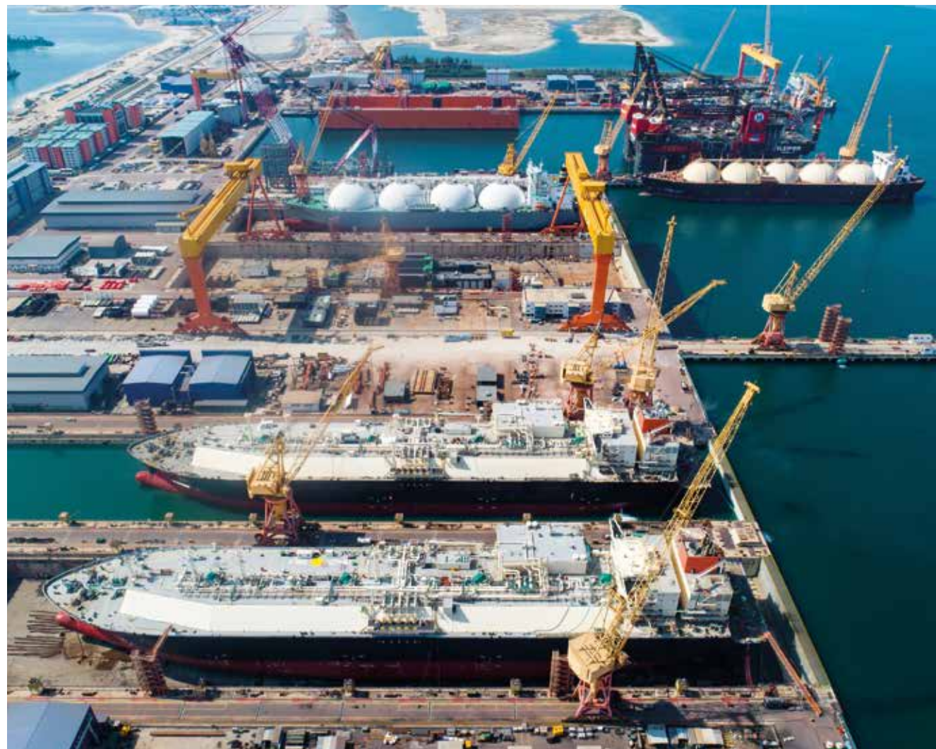
The Tuas Boulevard Yard strengthens Sembcorp Marine's value proposition as a one-stop solutions provider offering optimal production efficiency, cost-effective execution and shorter project delivery times
