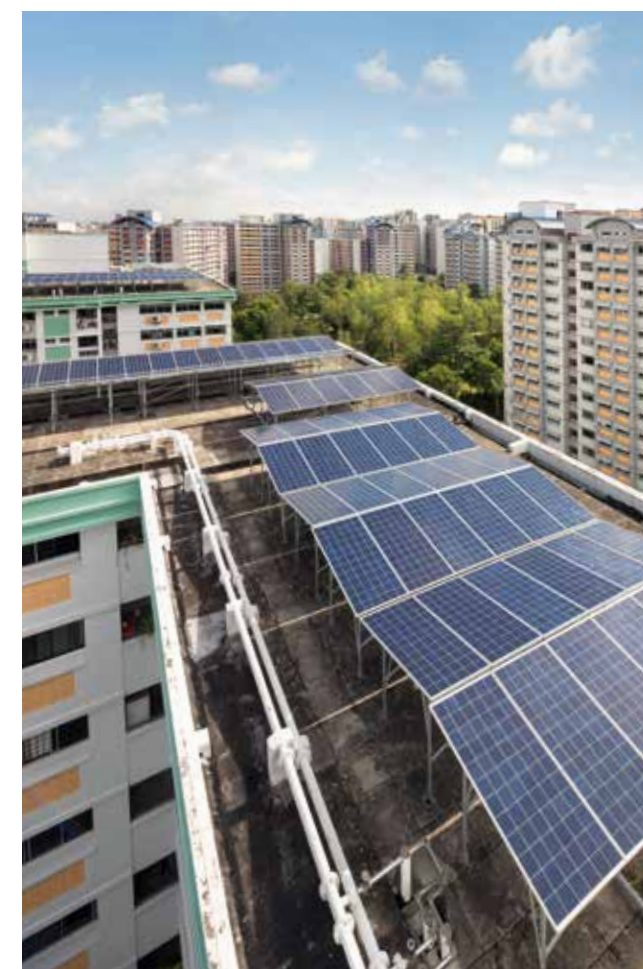
Sembcorp will build, own, operate and maintain grid-tied rooftop solar systems with a total capacity of 90 megawatt peak under the SolarNova programme
