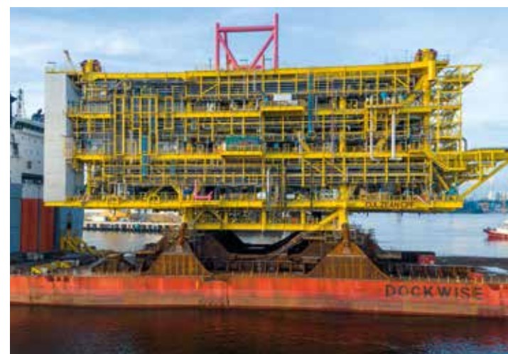
Delivered to TOTAL, this project involved the construction of wellhead, utilities and living quarters as well as central processing facility (pictured), for deployment in the Culzean field in the UK North Sea
