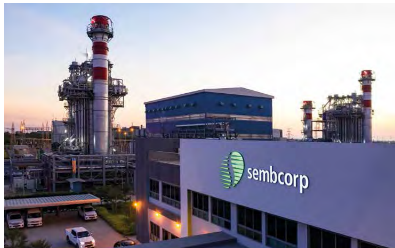
Sembcorp Myingyan Independent Power Plant will help to ease Myanmar’s power deficit
