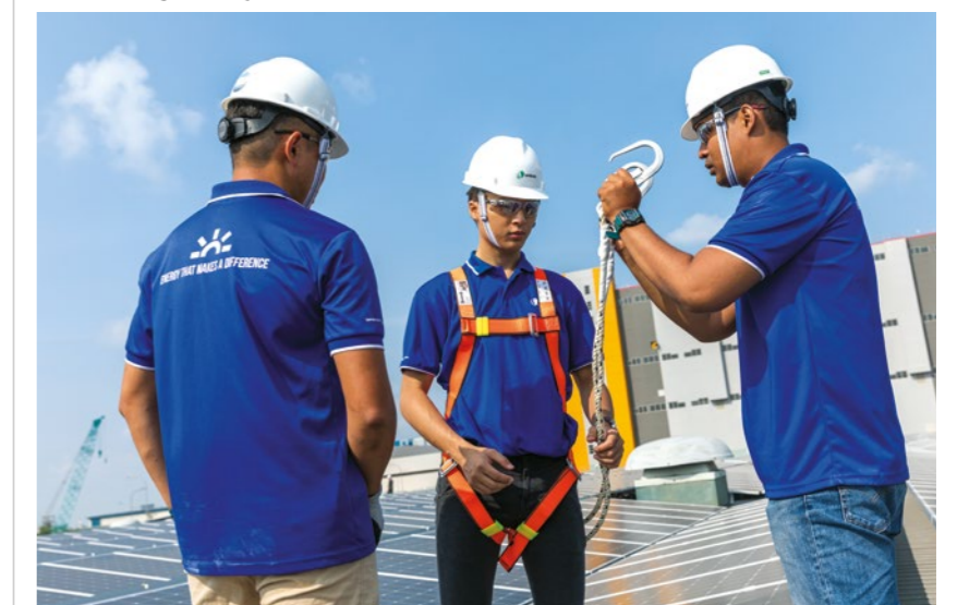
Sembcorp Solar safety personnel demonstrating the use of safety equipment
