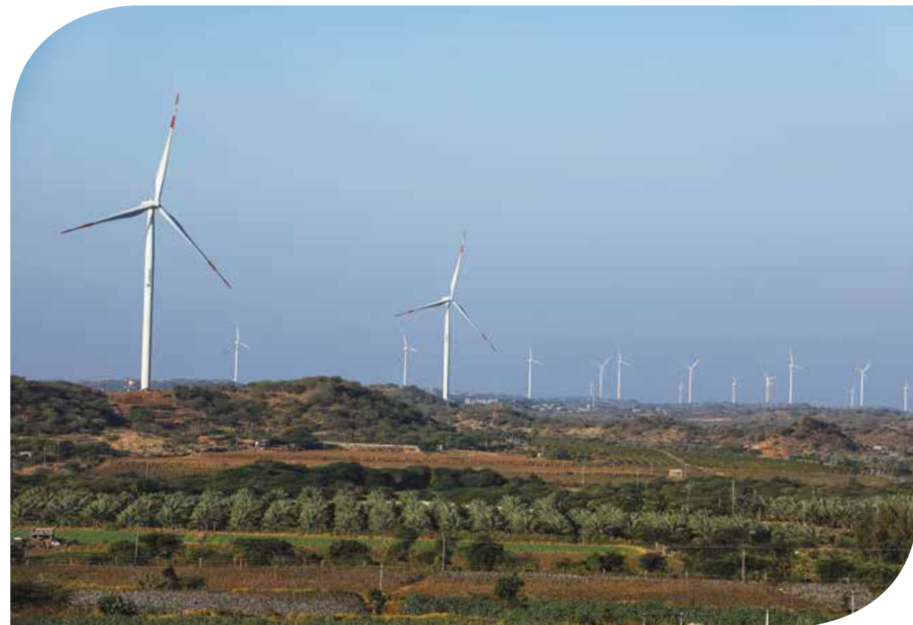
We secured a 400MW solar project in the Solar Energy Corporation of India (SECI) auction and fully commissioned our SECI 2 and SECI 3 wind projects – becoming the first independent power producer to complete projects awarded in the SECI 1, 2 and 3 tenders in India
