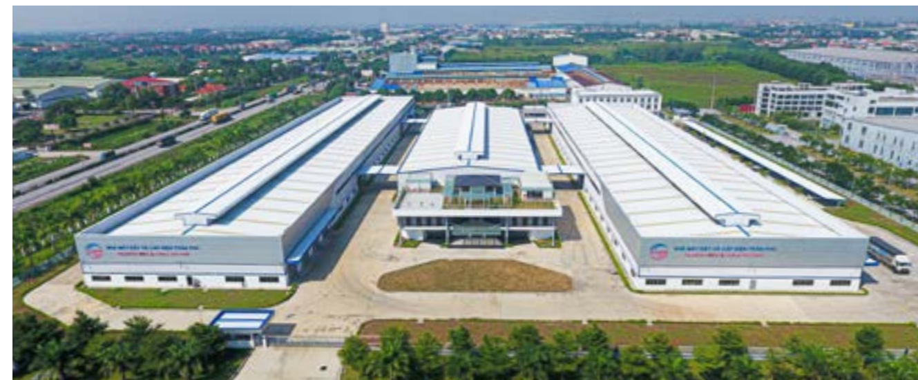
>> Tran Phu Wire & Cable Factory in VSIP Hai Duong
