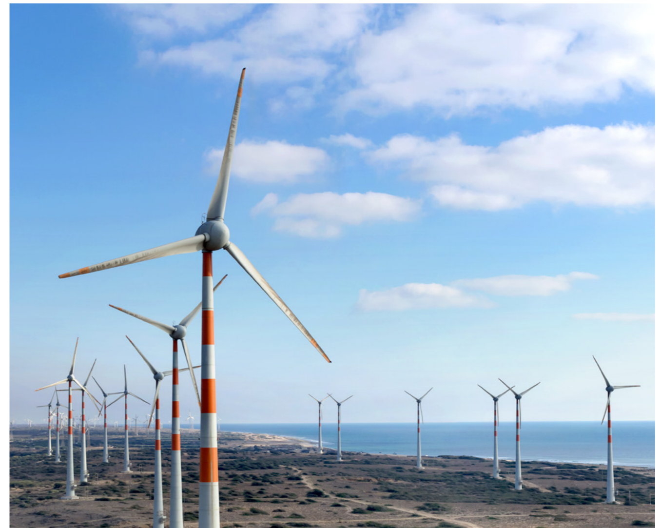
>> Sembcorp's wind power assets in Gujarat, India
