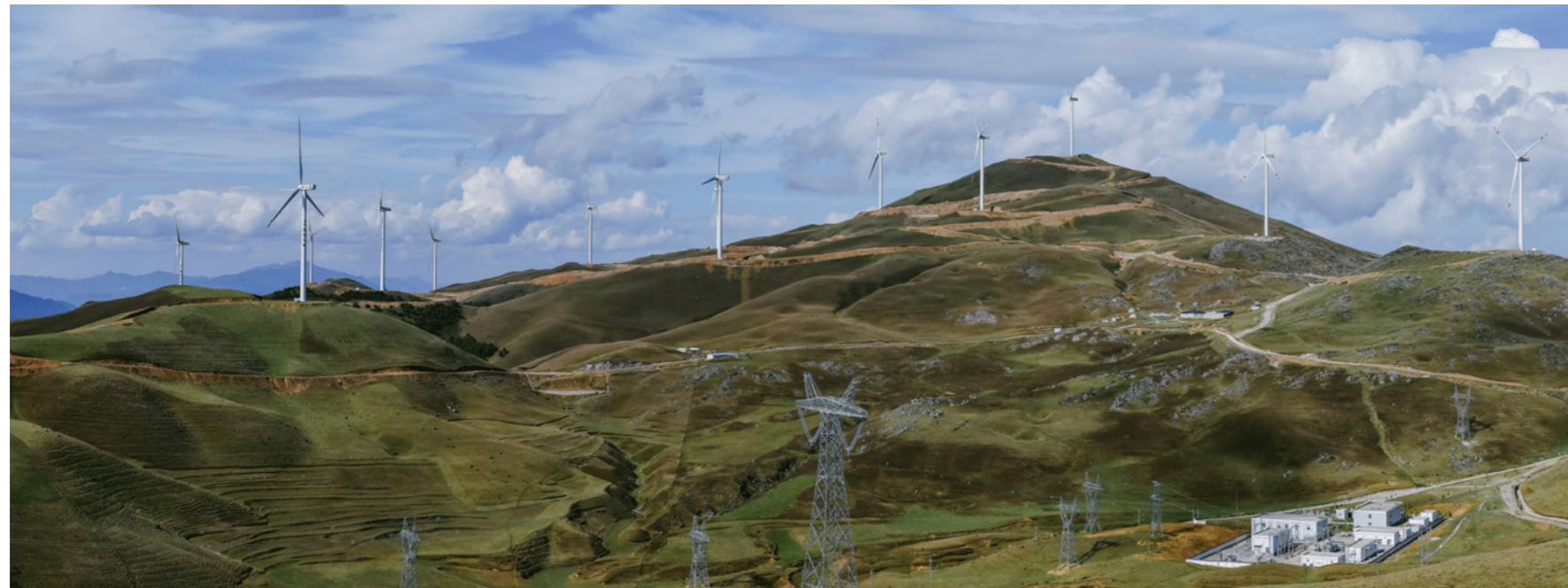
>> Wind assets in Yunnan province, China, jointly owned by Sembcorp and SDIC New Energy
