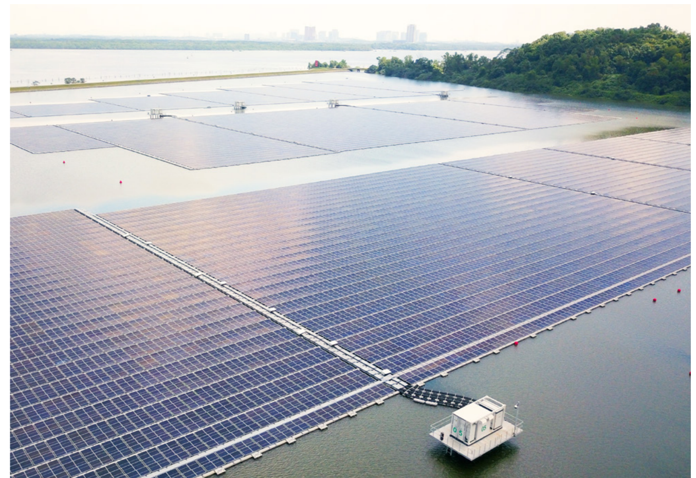
>> The 60MWp Sembcorp Tengeh Floating Solar Farm in Singapore, one of the largest inland floating solar farms in the world
