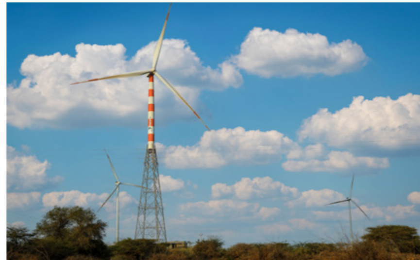
Sembcorp's wind power assets in Gujarat, India
