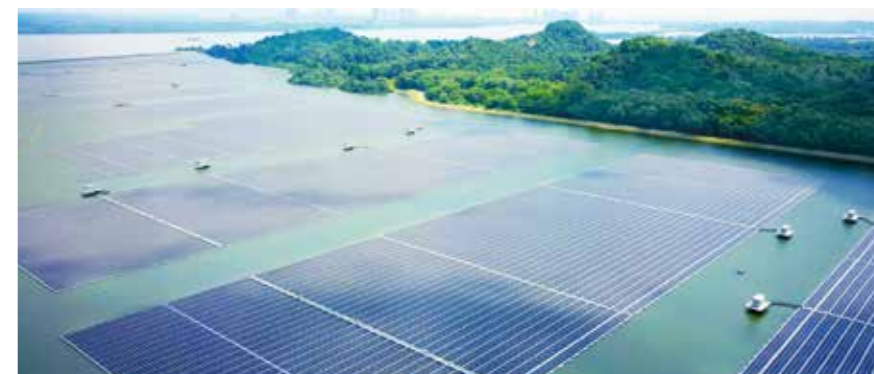
Sembcorp Tengoh Floating Solar Farm in Singapore
