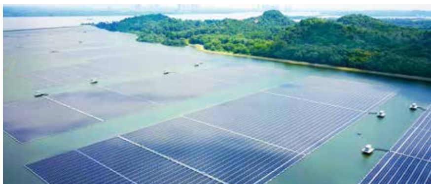
Sembcorp Tengoh Floating Solar Farm in Singapore
