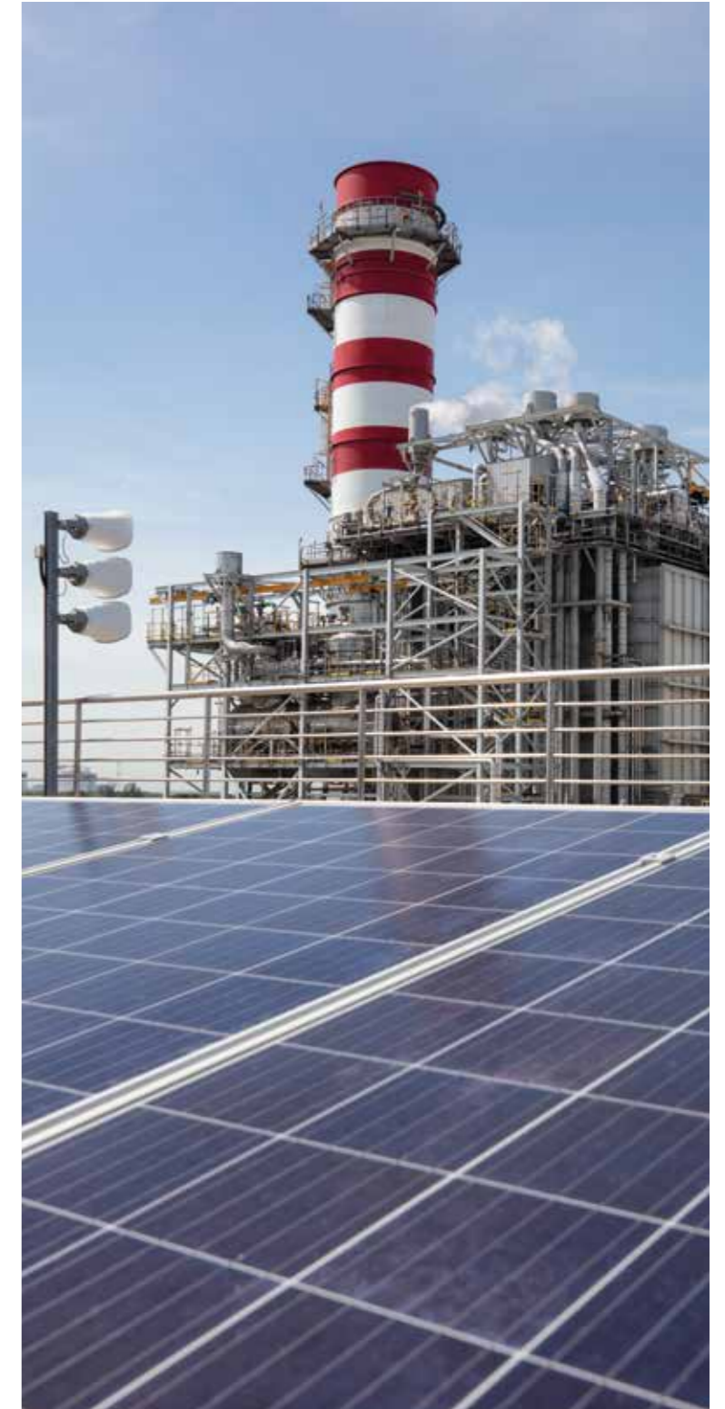
Sembcorp Cogeneration Plant, Banyan and solar panels installed on the rooftop of one of Sembcorp's facilities on Jurong Island, Singapore
