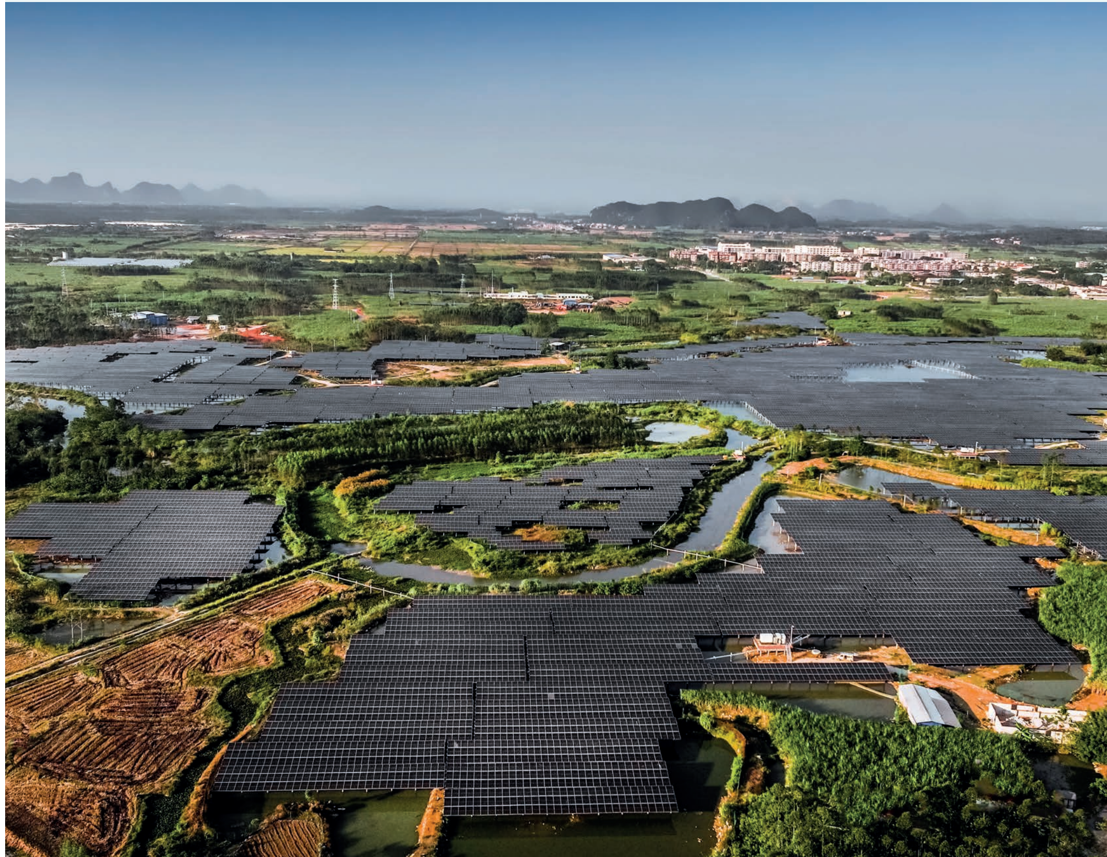
Sembcorp's solar assets in Guangxi, China
