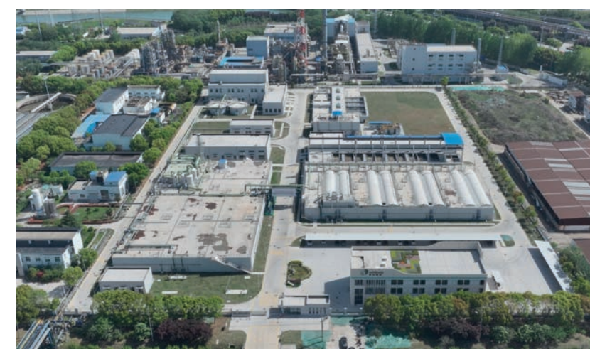
Sembcorp Nanjing Suiwu Wastewater Treatment Plant, China
