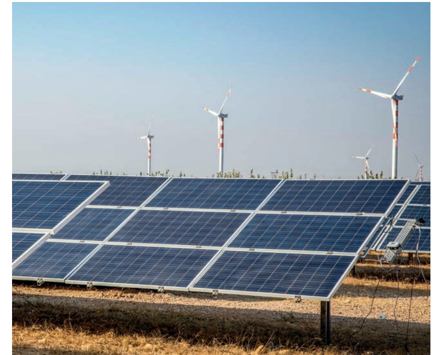
Sembcorp's hybrid renewables project in Rajasthan, India
