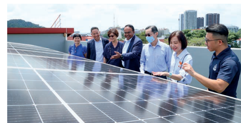
Representatives from Sembcorp, Community Foundation of Singapore and Boys' Town being briefed on the solarisation programme by Dr Roland Yeow, Executive Director of Boys' Town (far right)
