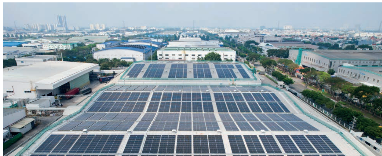
Rooftop solar panels installed on a tenant facility in Vietnam Singapore Industrial Park Binh Duong I, Vietnam
