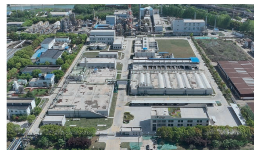
Sembcorp Nanjing Suiwu Wastewater Treatment Plant, China
