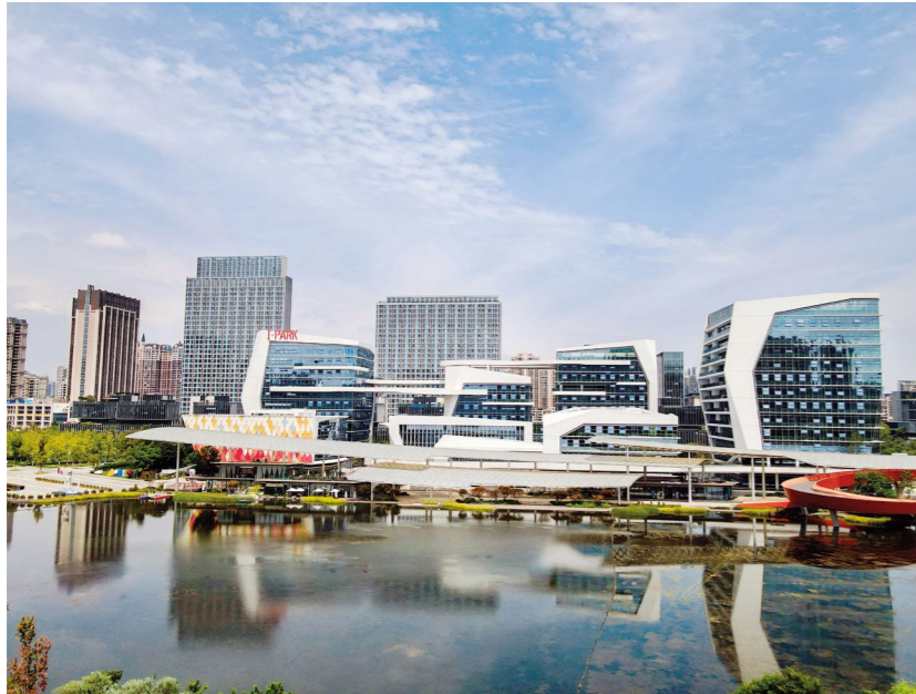
I-PARK Singapore Digital Innovation Park in Chengdu commenced operations in October 2025 and received healthy leasing enquiries
